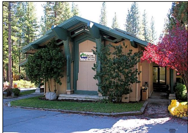
IVGID Administrative Offices
