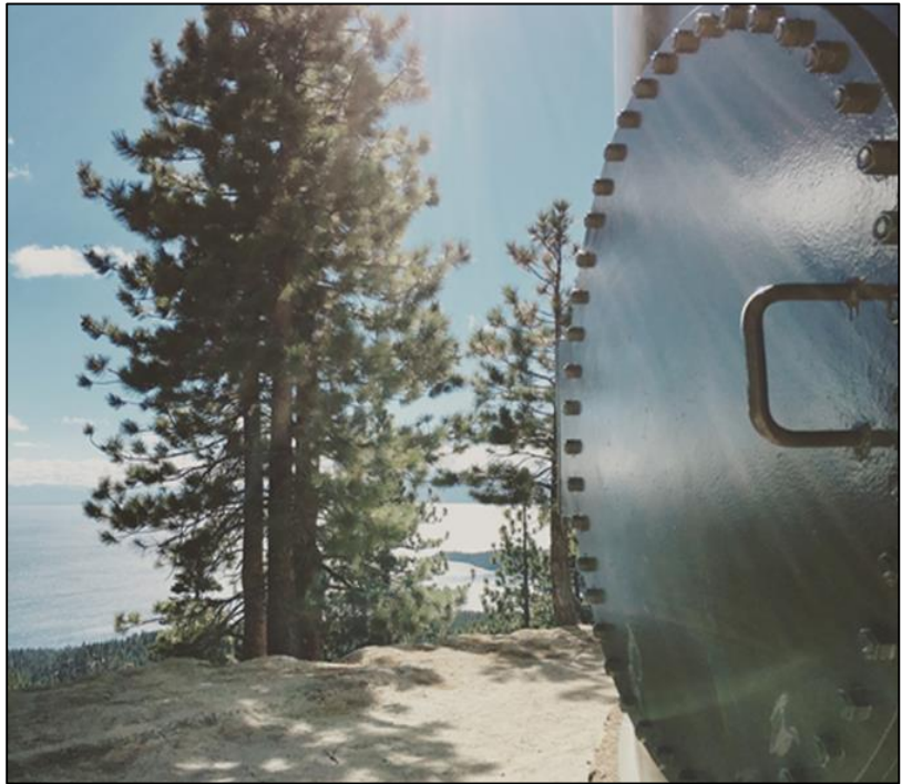
The upper-Tyner water tank (Reservoir 8-B1) is located at 7,771 feet in elevation and has a maximum drinking water capacity of 350,000 gallons.
