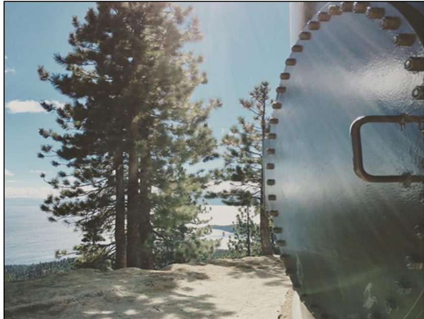
The upper-Tyner water tank (Reservoir 8-B1) is located at 7,771 feet in elevation and holds 350,000 gallons of drinking water.
