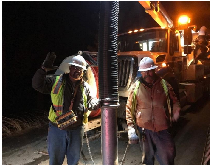
IVGID Public Works team members responding to an emergency
