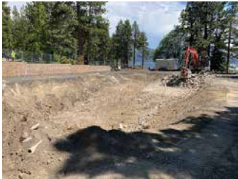
Pool Concrete Removal
