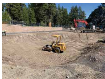
Old Pool Fill Compaction
