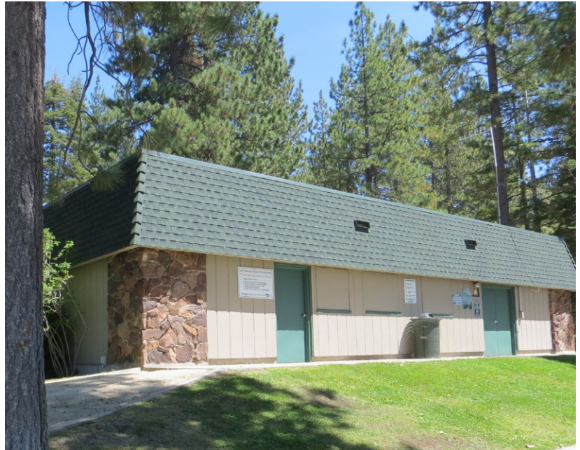
Key Idea: Replace Burnt Cedar Beach Restroom
