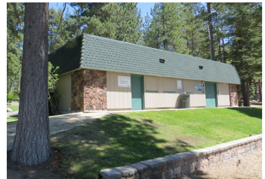
Burnt Cedar remote restroom and storage building
