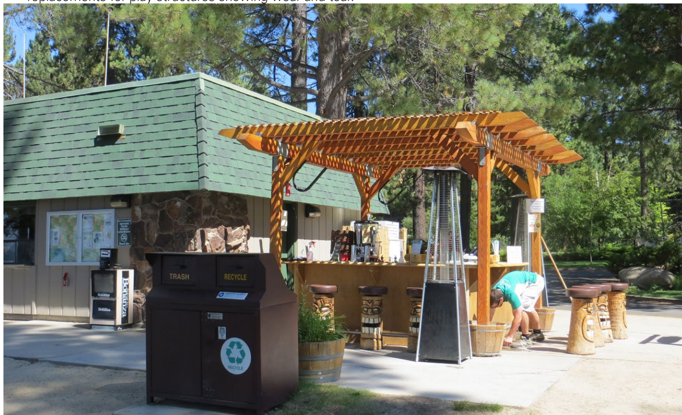
Replacement of the Incline Beach restroom is in the 2015-2016 CIP
