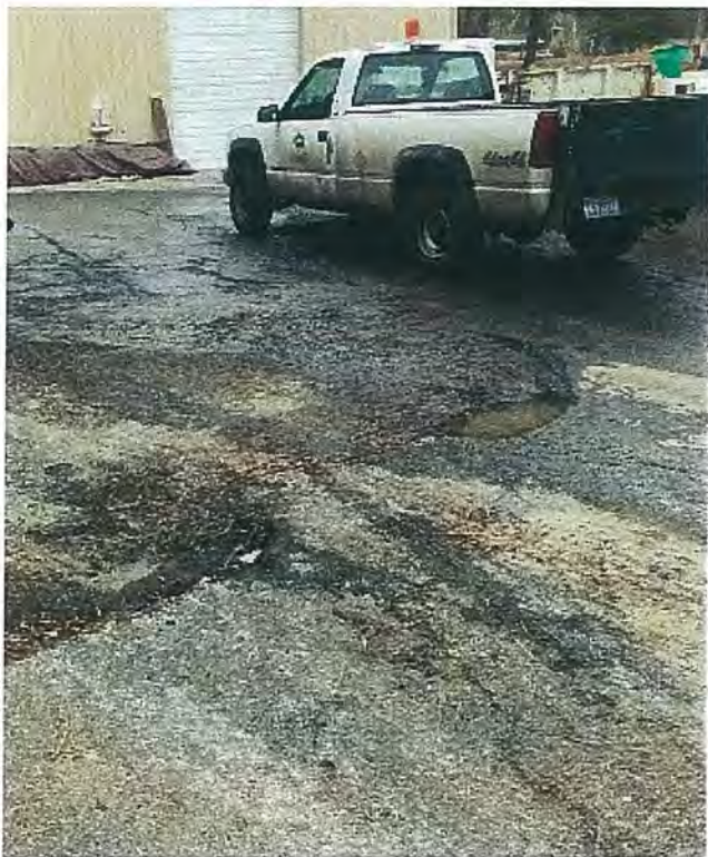
Photos 3 and 4. Deteriorated asphalt and existing stairs at Championship Maintenance Building.
