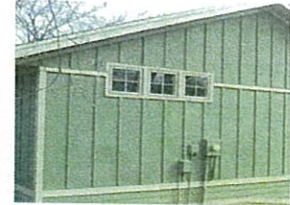
CONCRETE BOARD & BATTEN SIDING SCALE: 1/4" = 1'-0"
