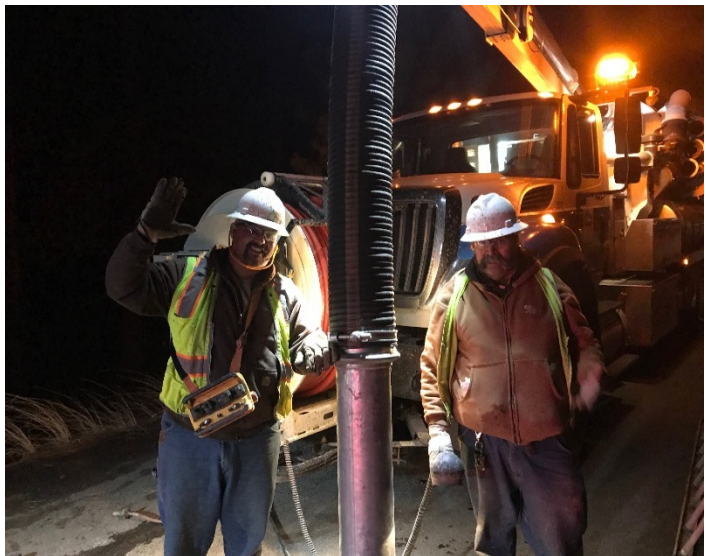
Chris and Alfie responding to a utility emergency
