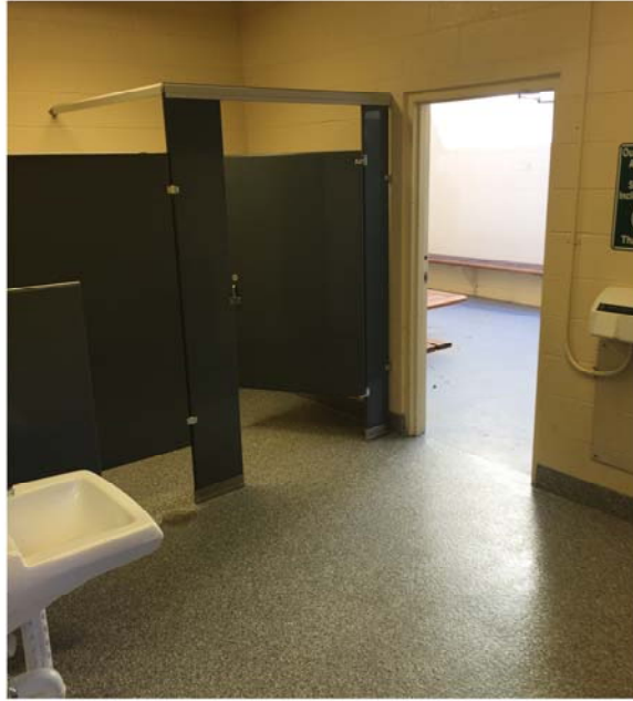
Buildings and Structures: Remote restrooms
