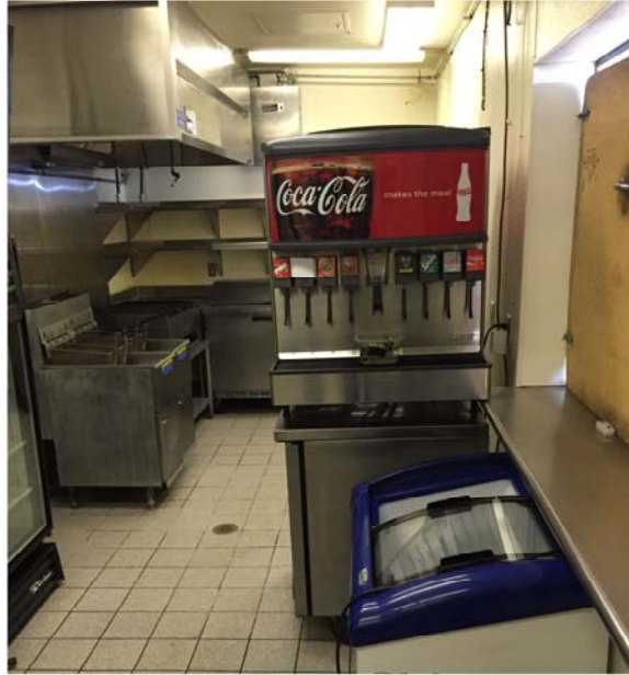
Buildings and Structures: Food Concessions
