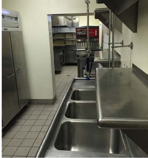
Buildings and Structures: Food Concessions
