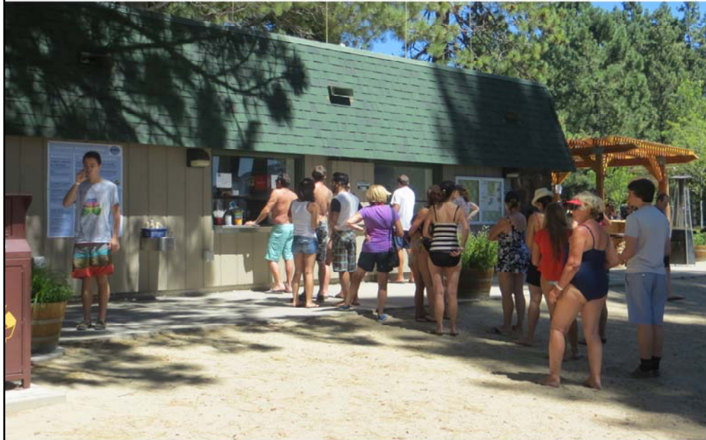
Buildings and Structures: Food Concessions
