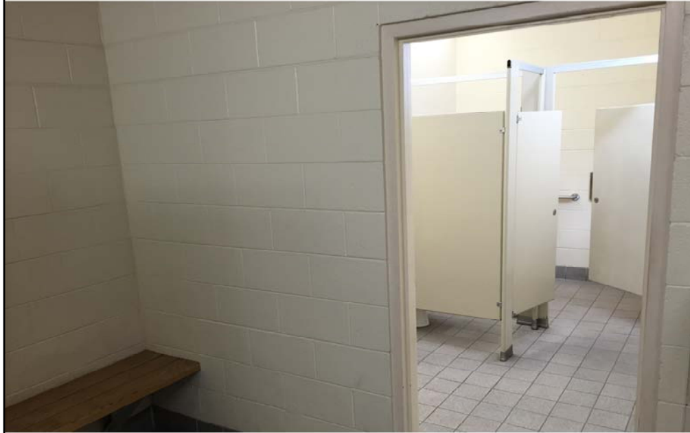
Buildings and Structures: Incline Beach restroom facilities
