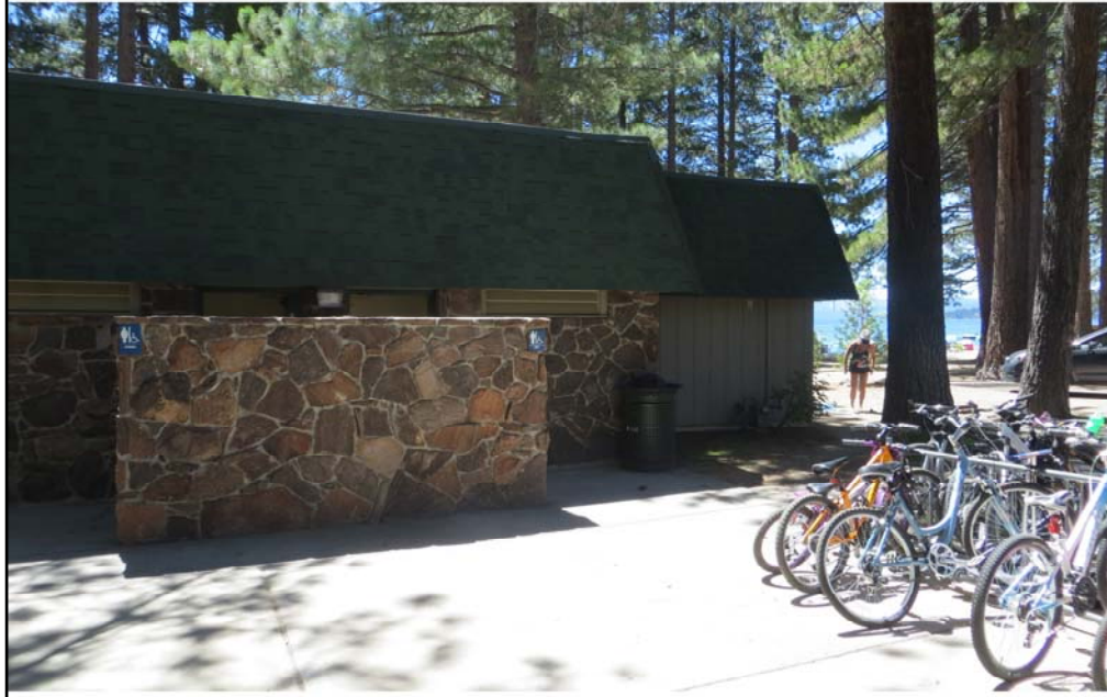
Buildings and Structures: Incline Beach restroom facilities
