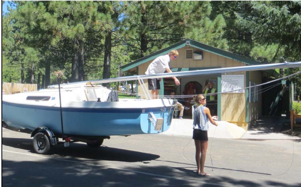
Buildings and Structures: Ski Beach restroom and storage facilities
