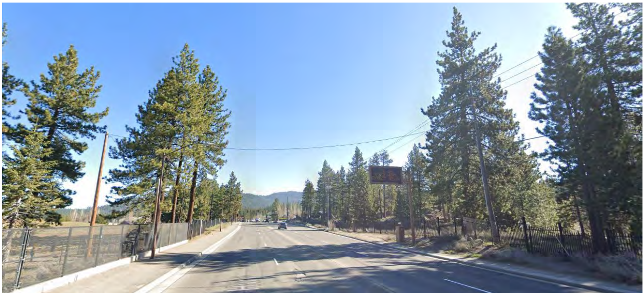
Figure 51: Power poles along US 50 crossing Edgewood Creek in Stateline that are in or near a 100-year floodplain (Source: Google Street View, Apr 2019)
