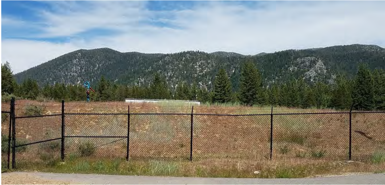
Figure 55. Levee at the STPUD wastewater treatment plant
