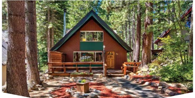
599 CREST LANE INCLINE VILLAGE
