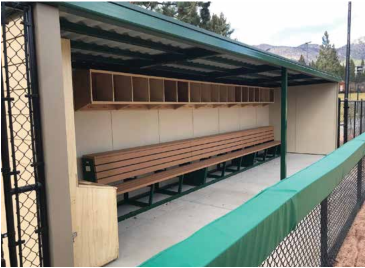
Incline Park Ballfield Renovations
