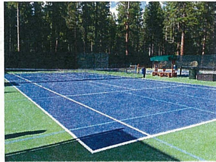
IVGID Tennis Court #10 Pickleball & Tennis striping
