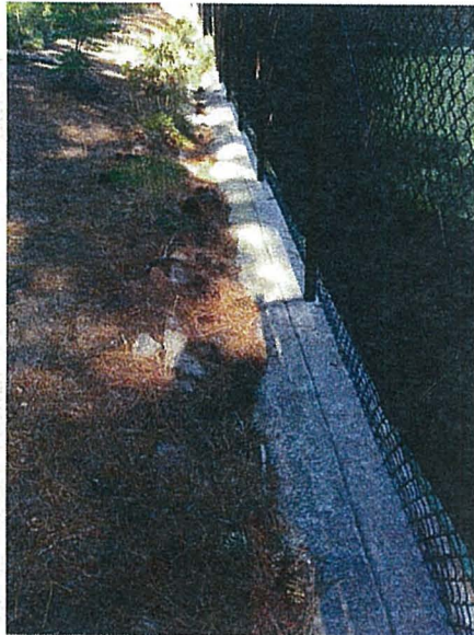
Court V-Drain maintenance
