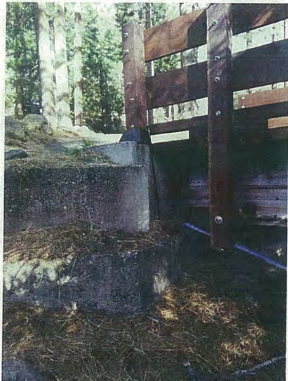
Photo 16 – View of West Abutment
