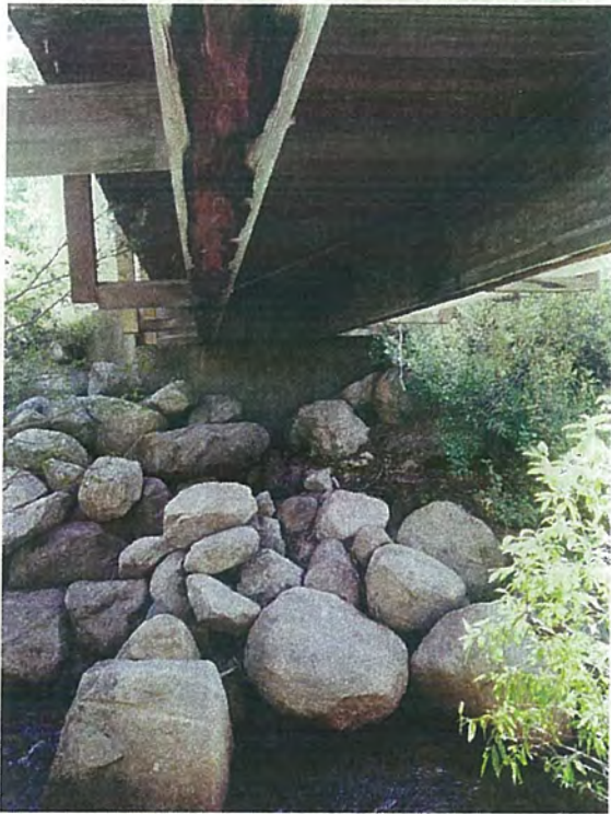
Photo 13 – View of Northeast Abutment
