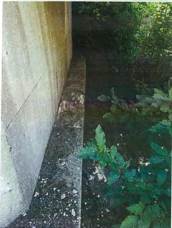
Photo 25 – View of North Abutment
