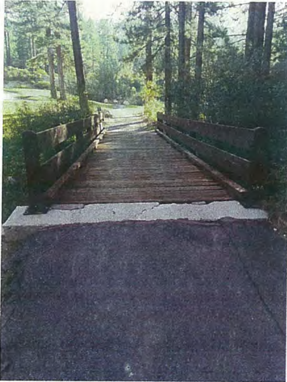
Photo 1 – Bridge Looking East
