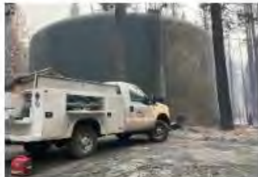
The 2021 Caldor Fire nearly devastated the Arrowhead Tank. Photo by South Tahoe Public Utility District.
