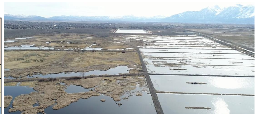
IVGID Wetlands Enhancement Facility in Carson Valley, NV
