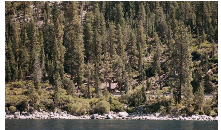
The IVGID Spooner Pump Station (effluent export line pump) blends into its surroundings along Highway 28, south of Sand Harbor Nevada State Park
