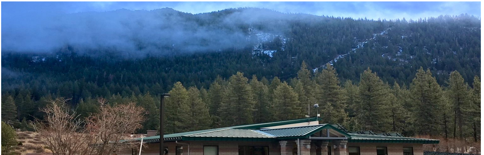
IVGID Public Works Facility located at 1220 Sweetwater Road in Incline Village, NV
