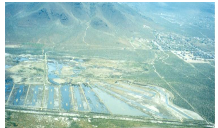
IVGID Wetlands Enhancement Facility in Carson Valley, NV
