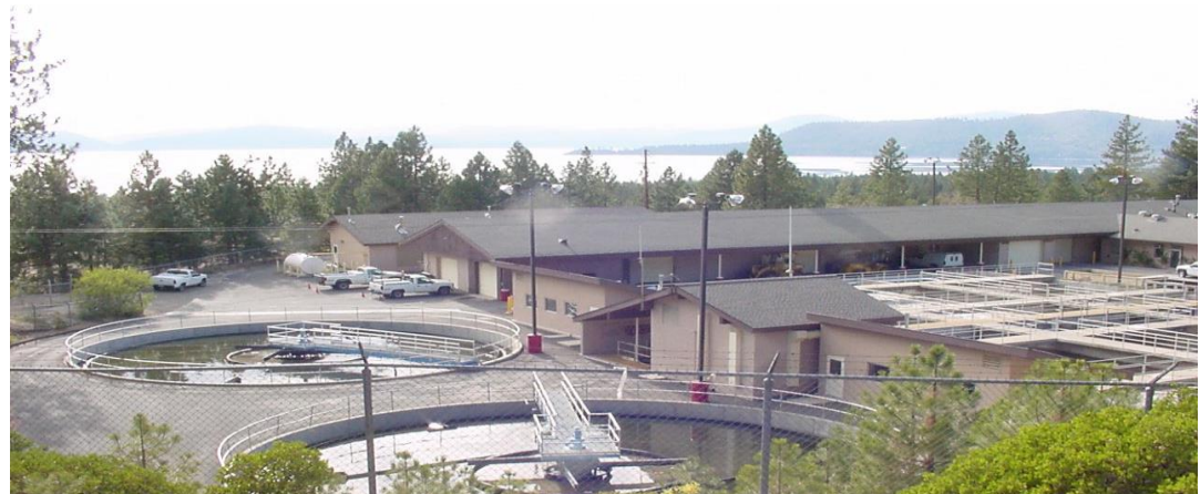
Water Resource Recovery Facility (WRRF) located at 1250 Sweetwater Road in Incline Village, NV
