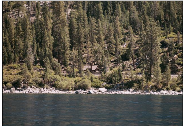
The Spooner Pump Station along Highway 28 blends into its surroundings.
