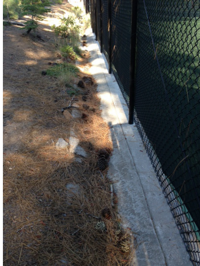
Court V-Drain maintenance
