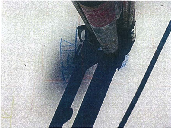
Pool Photo #7 Coring machine on swimming pool floor.
