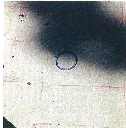
Pool Photo #6 Mapping of core location at swimming pool floor. Note additional mapping of rebar.
