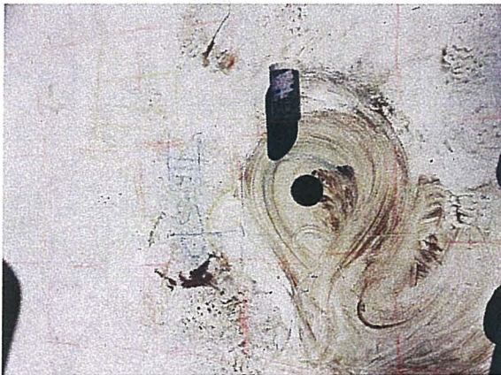
Pool Photo #9 Cored hole in swimming pool floor. Note, core sample for additional compression strength testing.
