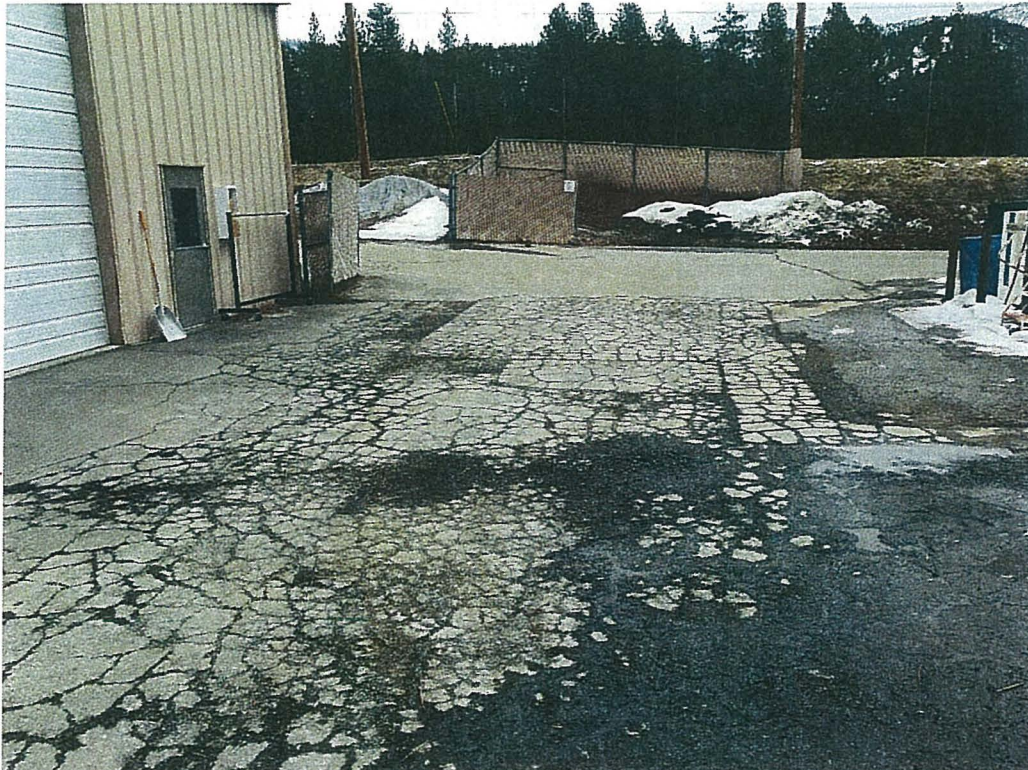
Photo 5. Deteriorated asphalt proposed to be replaced as part of a change order.
