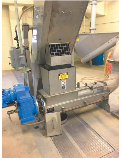
Figure 49: Example Screen (Debris Washer/Compactor)
