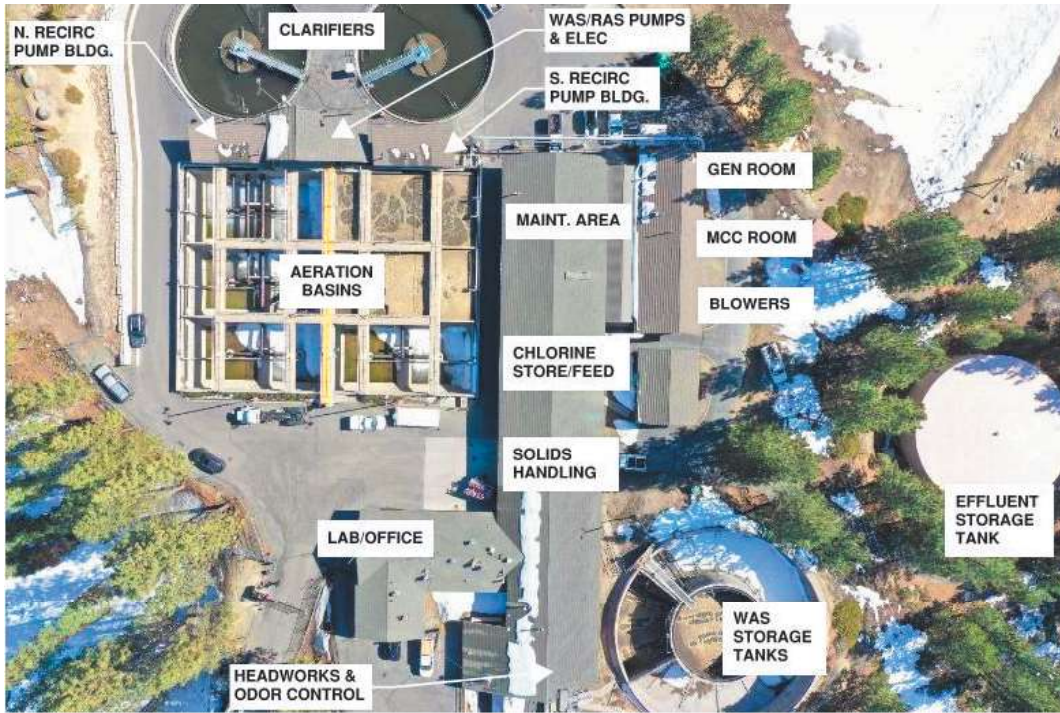
Figure 25: Water Resource Recovery Facility–Site Overview
