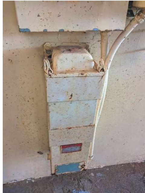
Figure 85: Transformer Corrosion
