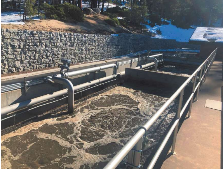
Figure 53: North Aeration Basins, Under Aeration (N-2, N-3)
