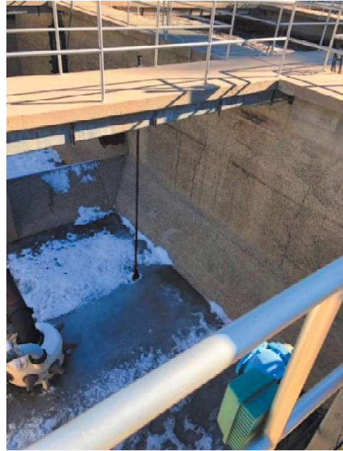
Figure 61: Aeration Basin Concrete
