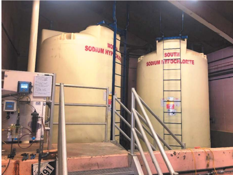
Figure 72: Hypochlorite Tanks
