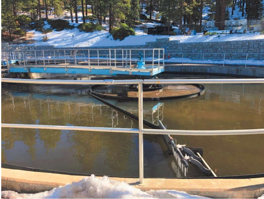
Figure 69: Secondary Clarifier
