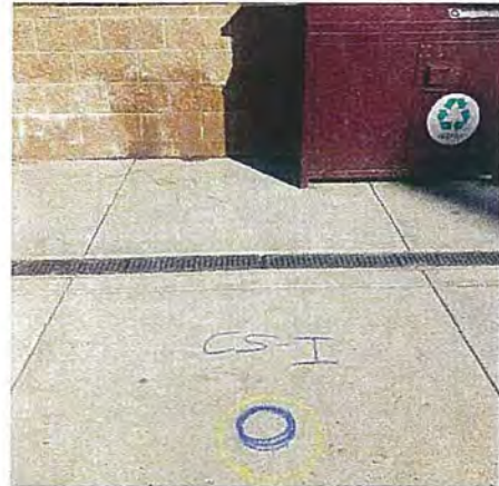
Pool Photo #4 Mapping of core locations on pool deck.
