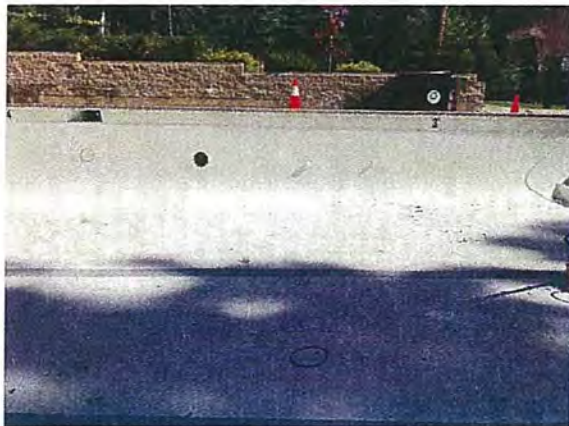
Pool Photo #5 Mapping of core locations on swimming Pool floor.
