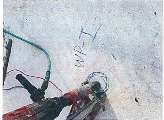
Pool Photo #8 Coring machine on wading pool floor.
