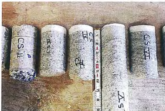
Pool Photo #11 Close-up of core samples. Note relative thickness of concrete cores.
